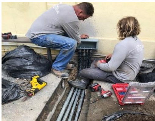
Trenching and electrical installation between the Parish Hall & Sanctuary
