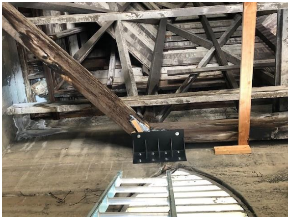
Bell Tower Repairs
