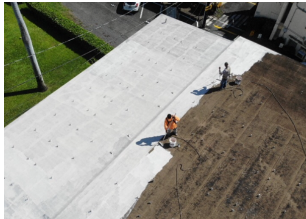
Primer coating being rolled on the Parish Hall roof
